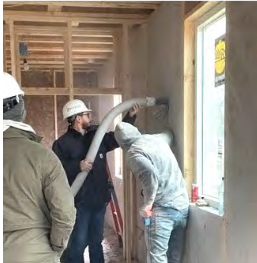
Students helping with cellulose installation
