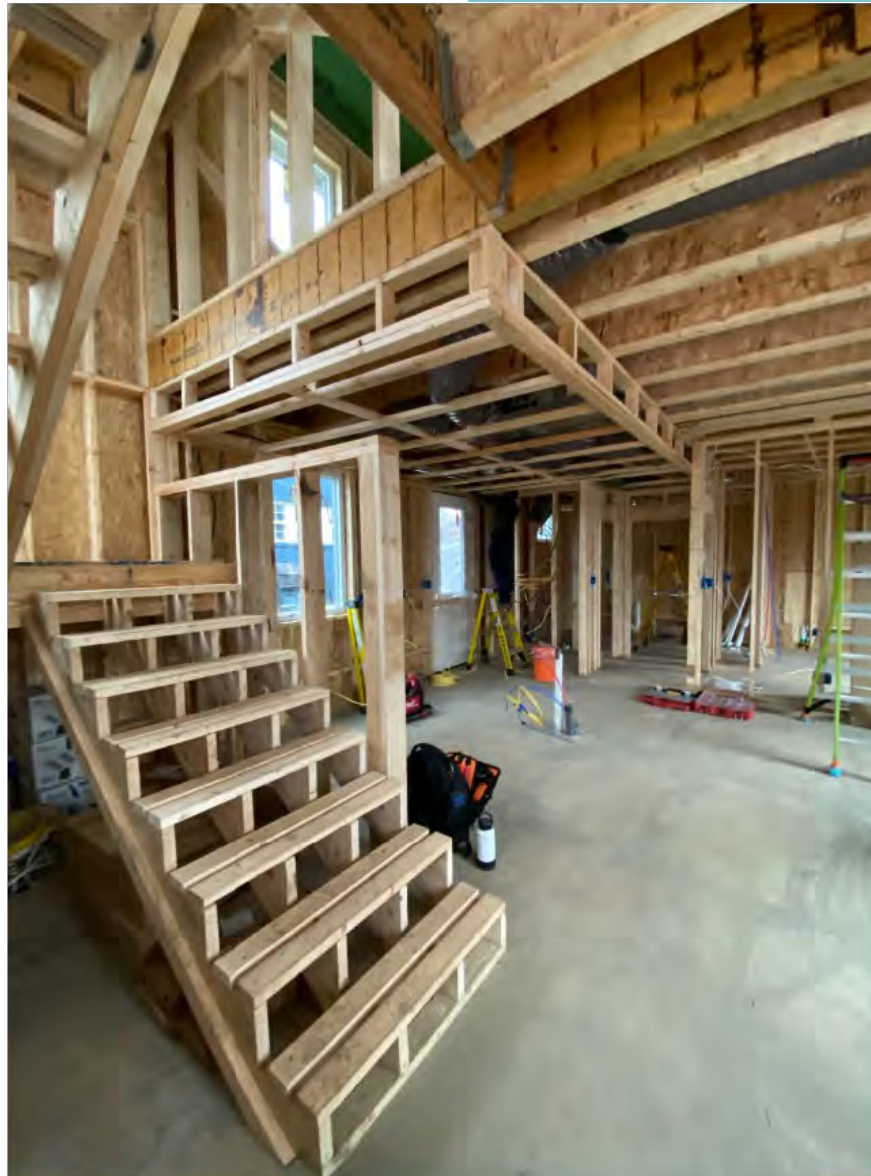
First Floor Framing
