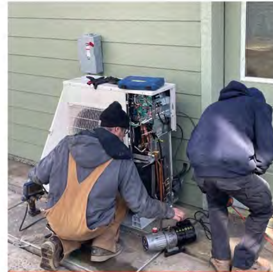
Outdoor Heat Pump Install
