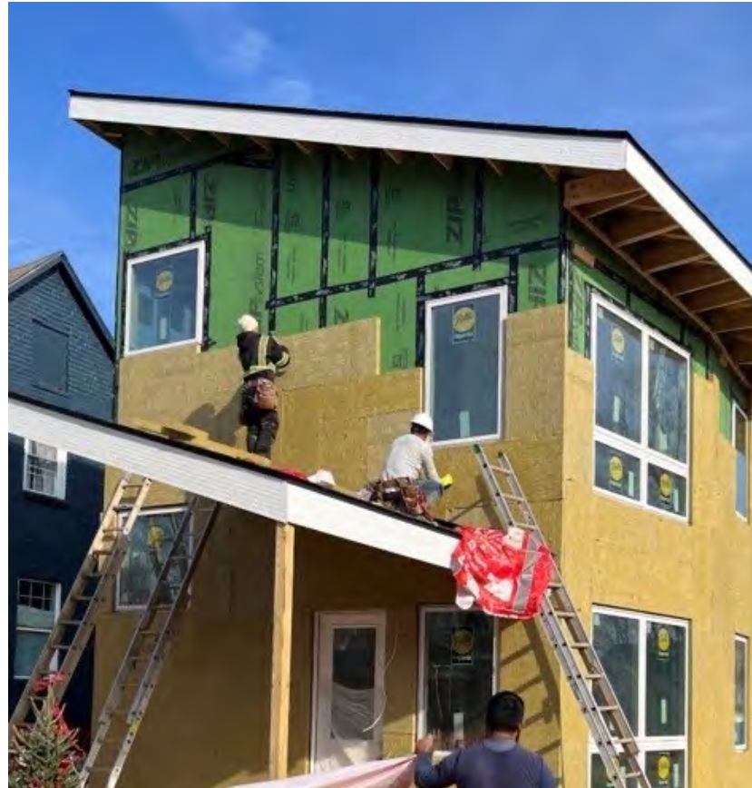
Installation of two layers of Rockwool
